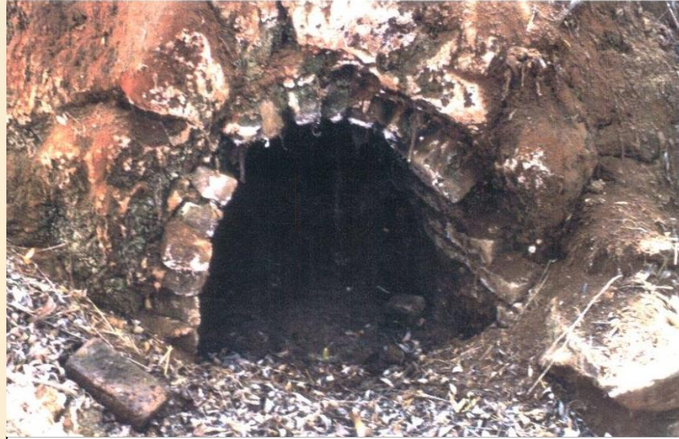
Access arch of the Bell Canyon limekiln 1987 photo courtesy Leonis Adobe The bricks in the access arch are not adobe bricks, but fired bricks from the 1850s-60s American Period.
